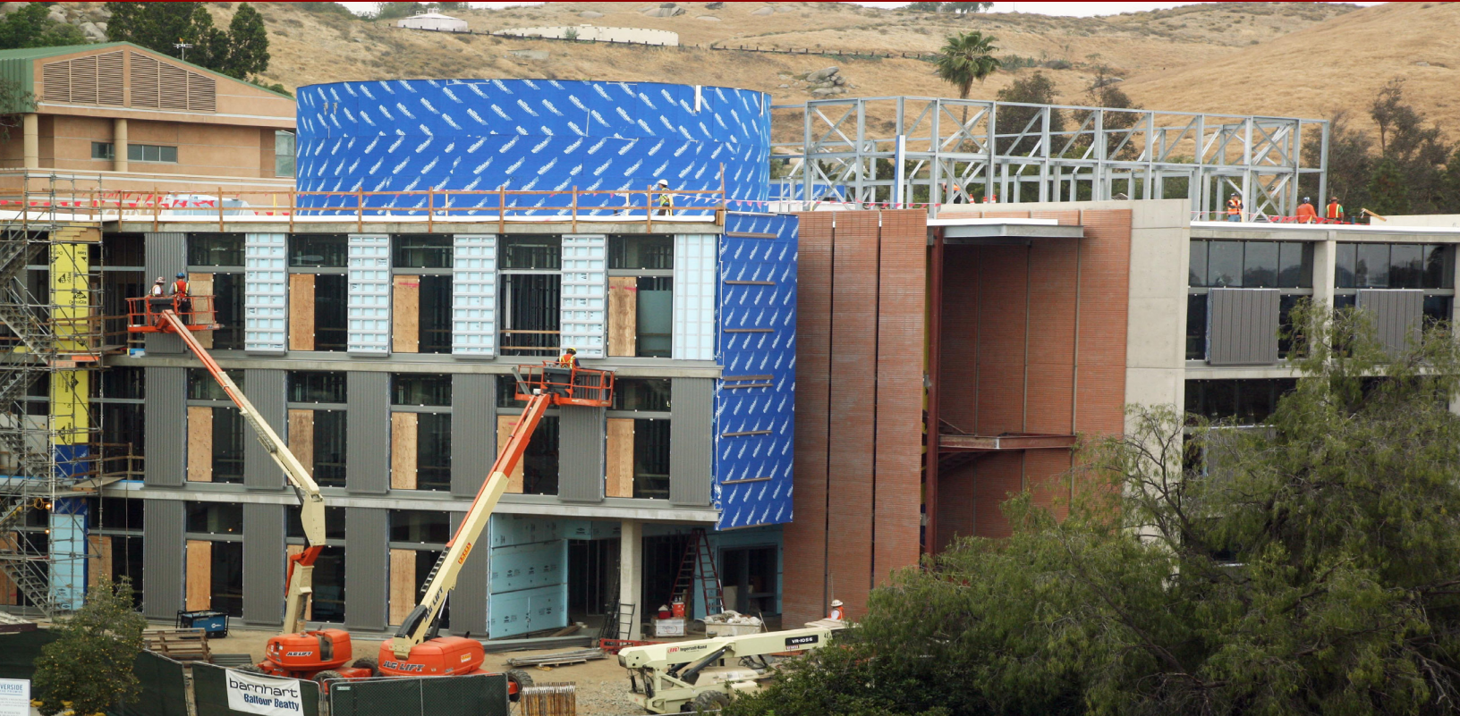
PHOTO: CONSTRUCTION OF THE UCR HEALTH SCIENCES RESEARCH BUILDING
